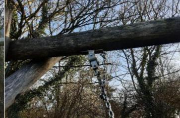
**Finding:** A number of fixing(s) have worked loose on the suspension mounts. The office and client have been notified of this
