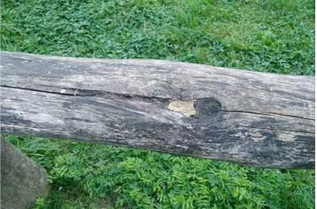
**Finding:** The use of synthetic fillers in timber is not recommended; timber being a natural material will expand and contract as the moisture content changes and the use of fillers can exacerbate the length and depth of these cracks or shakes in the timber. The only treatment that is normally required is the removal of any rough or sharp edges unless the structural integrity of the item is affected.
