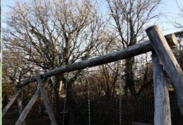
**Action:** We would recommend that the joint be dismantled and checked on a regular basis or consulting with manufacturer on whether a Secondary Safety Device can be fitted
