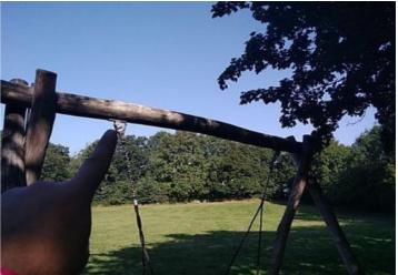
**Finding:** A number of fixing(s) have worked loose on the secondary safety chain
