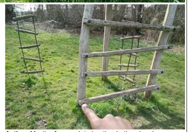
Finding: There is some damage apparent on the posts, this Action: Monitor for any deterioration (rot) and replace as can penetrate the preservative applied to the timber and accelerate the rotting process
