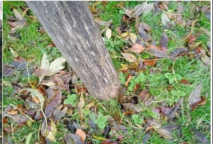
**Finding:** There is some strimmer / machinery damage apparent on the posts, this can penetrate the preservative applied to the timber and accelerate the rotting process. **Action:** Monitor for any deterioration (rot) and replace as required
