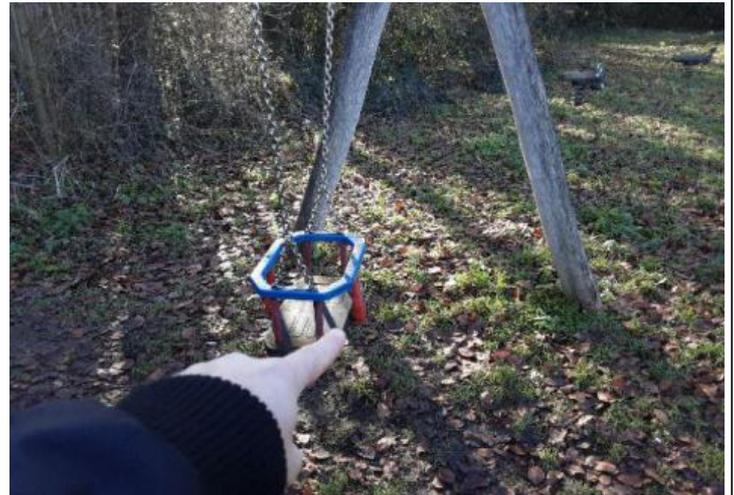
**Finding:** The swing seat frame is severely corroded and requires replacement
