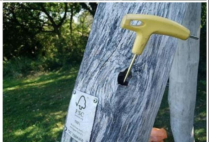
**Finding:** There is a large cavity within the timber support and the inspector has some concerns about the internal condition of the timber and was unable to verify the structural integrity without further testing. We recommend a Resi-PD survey to establish the condition of the timber at it's core.
