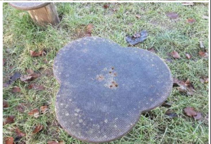
**Finding:** The platforms are rotting and the fixings are pulling through
