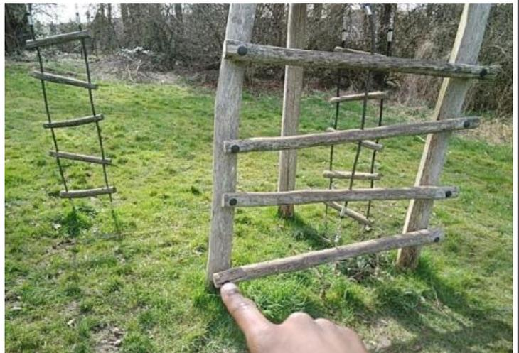
**Finding:** There is some damage apparent on the posts, this can penetrate the preservative applied to the timber and accelerate the rotting process
