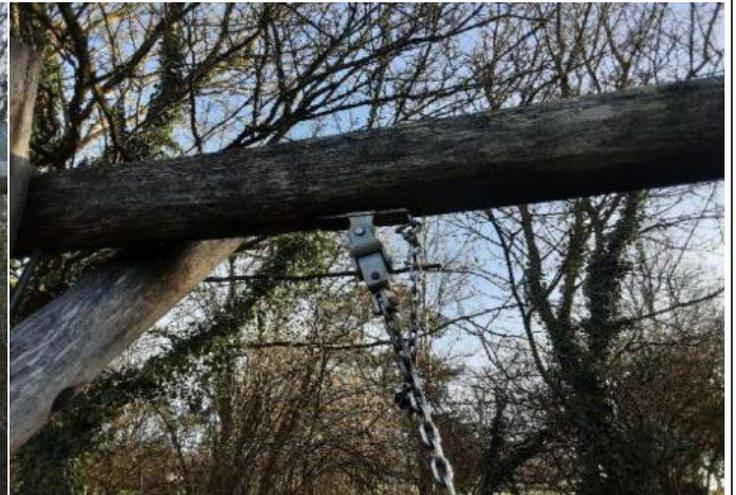
**Finding:** A number of fixing(s) have worked loose on the suspension mounts
