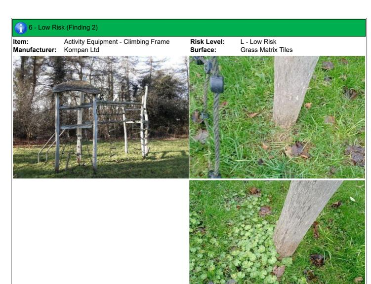
**Finding:** There is some strimmer / machinery damage apparent on the posts, this can penetrate the preservative applied to the timber and accelerate the rotting process
