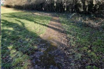
**Finding:** There is algae, silt or moss growth on the pathway **Action:** Clean and treat appropriately surface resulting in slippery conditions
