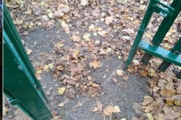
**Finding:** The gate has no drop bolt sleeves and/or drop bolts fitted
