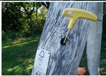
**Finding:** There is a large cavity within the timber support and the inspector has some concerns about the internal condition of the timber and was unable to verify the structural integrity without further testing. We recommend a Resi-PD survey to establish the condition of the timber at it's core.
