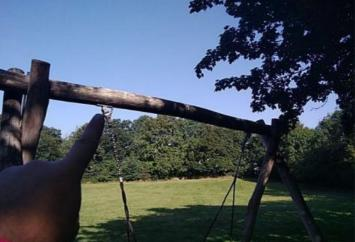
**Finding:** A number of fixing(s) have worked loose on the secondary safety chain
