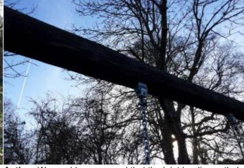
Action: We would recommend that the joint be dismantled and checked on a regular basis or consulting with manufacturer on whether a Secondary Safety Device can be fitted
