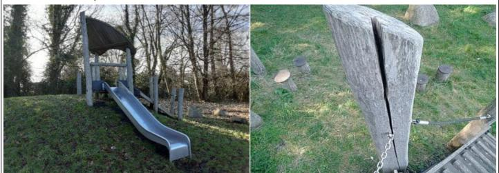
**Finding:** The timber has a number of splits/shakes or air **Action:** Monitor to ensure the splits do not cross through cracks and this may affect the stability or allow water ingress fixing points of the structure and/or cause any instability which will accelerate the rotting process
