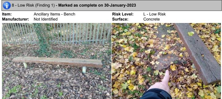
Finding: There are trip hazards at the edges of the surface Action: Reinstate surrounding surface levels to remove the trip points
