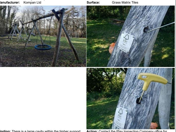
**Finding:** There is a large cavity within the timber support and the inspector has some concerns about the internal condition of the timber and was unable to verify the structural integrity without further testing. We recommend a Resi-PD survey to establish the condition of the timber at it's core.
