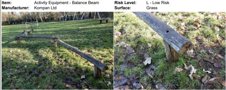
**Finding:** The timber has a number of splits/shakes or air cracks and this may affect the stability or allow water ingress fixing points of the structure and/or cause any instability which will accelerate the rotting process
