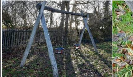
**Finding:** There is some strimmer / machinery damage apparent on the posts, this can penetrate the preservative applied to the timber and accelerate the rotting process
