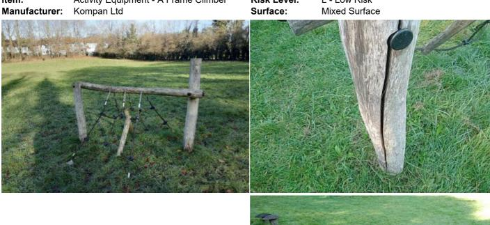
Finding: The timber has a number of splits/shakes or air Action: Monitor to ensure the splits do not cross through cracks and this may affect the stability or allow water ingress fixing points of the structure and/or cause any instability which will accelerate the rotting process
