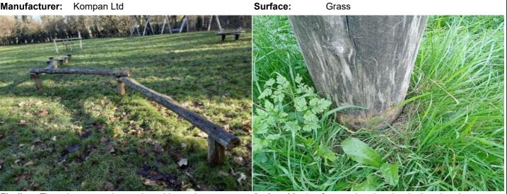
**Finding:** There is some strimmer / machinery damage apparent on the posts, this can penetrate the preservative applied to the timber and accelerate the rotting process
