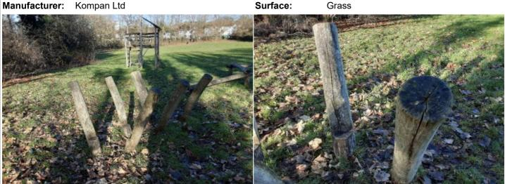
**Finding:** The timber has a number of splits/shakes or air cracks and this may affect the stability or allow water ingress fixing points of the structure and/or cause any instability which will accelerate the rotting process
